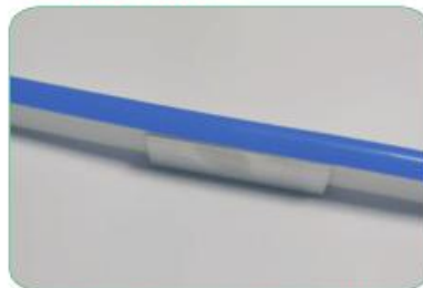
6 Fix the position with aluminum mountings
